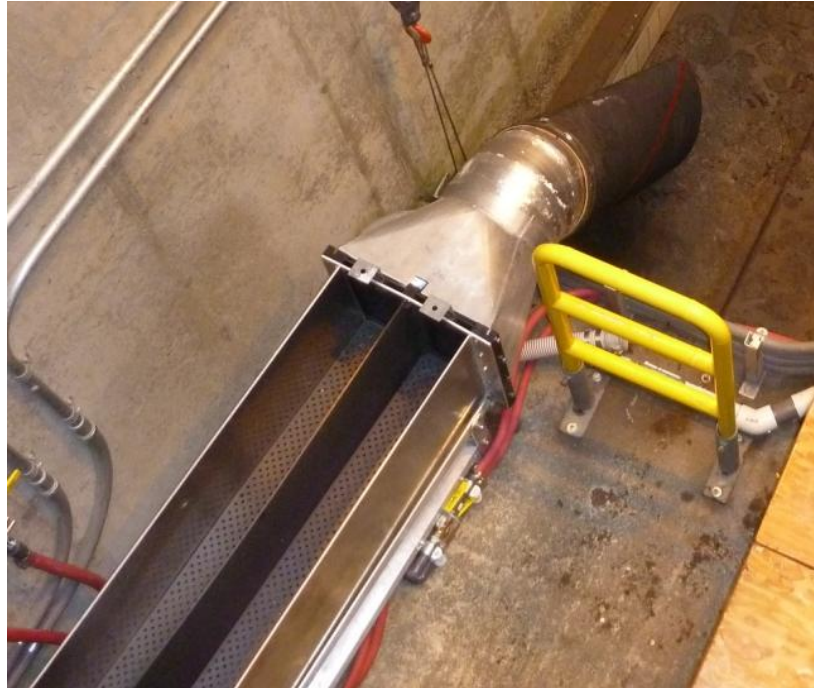
Figure 5: Observation and recovery tank with exit chute to brail pool.
