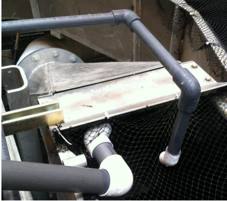
Figure 10: Additional water supply to north bypass flume (larger left pipe).
