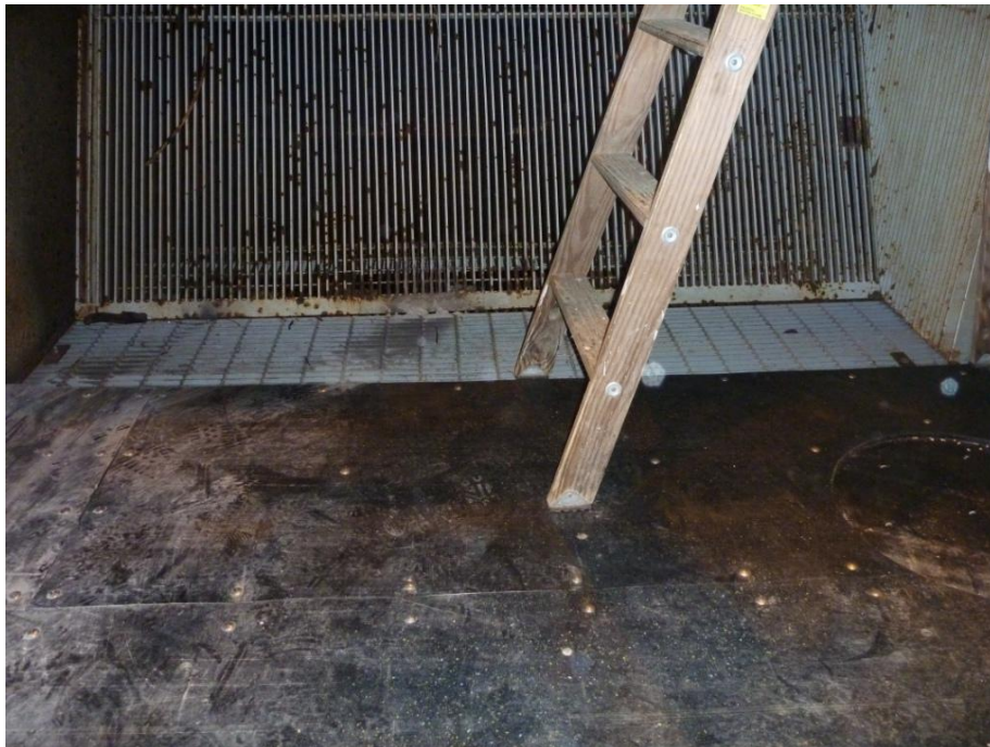
Figure 3: UHMW floor plating fastened to the return pool floor grating
