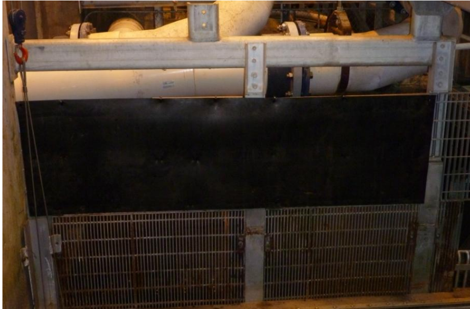
Figure 8: Brail pool fencing with new neoprene panel.
