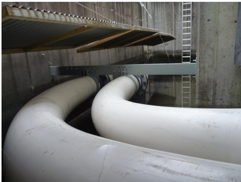
Figure 7: Extended bypass pipes outside the lab following installation.
